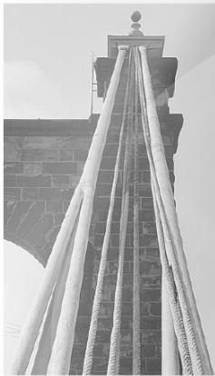
The main span is 1,010 feet (310 m) from tower to tower. The east tower rests on the Wheeling shore, while the west tower is on Wheeling Island. The east tower is 153.5 feet (46.8 m) above the low-water level of the river, or 82 feet (25 m) from the base of the masonry. The west tower is 132.75 feet (40.46 m) above low water, with 69 feet (21 m) of masonry. (6) Detailed analysis of the bridge has contributed to the life work of Dr. Emory Leland Kemp, Emory Kemp
