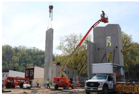
(Walls for the Hose Tower being assembled - view from Wood St.)
